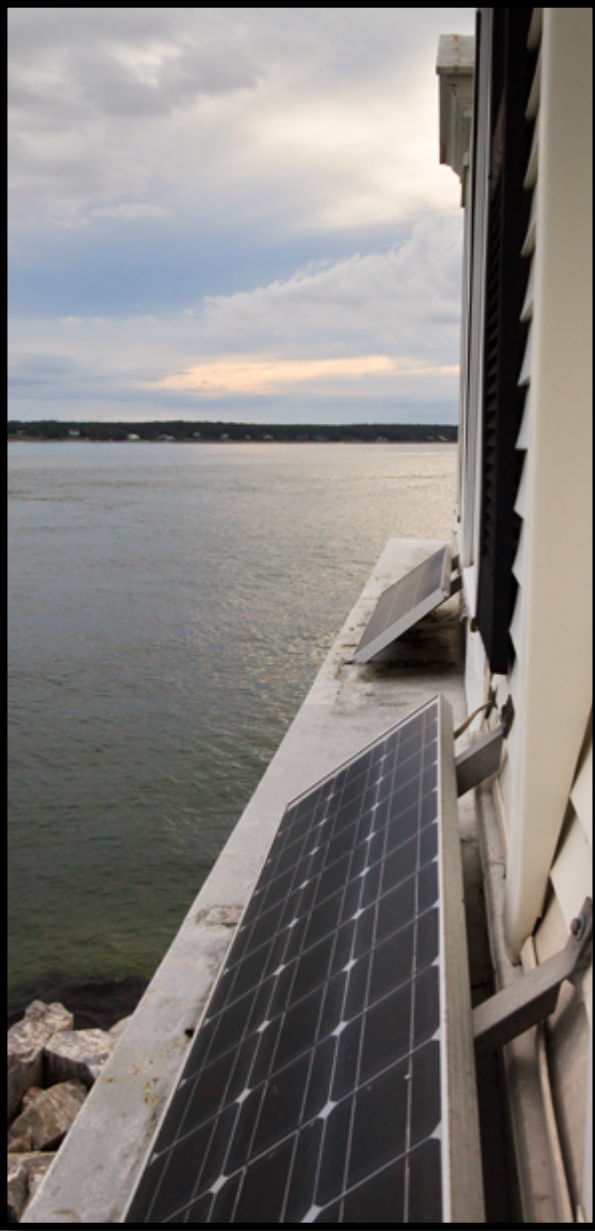
A closer look at the solar panels on the lower roof line that power the Light and structure.
